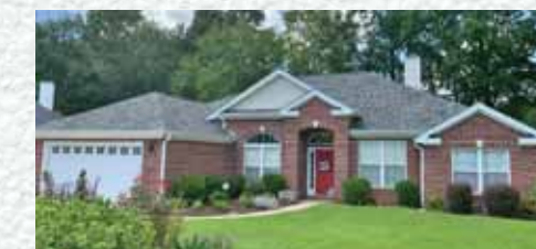
All American Management Group recently aligned itself with an established local roofing company which now gives the company the ability to be a true “turnkey” operation that can handle the majority of exterior product needs for the building contractors, property managers and homeowners.
