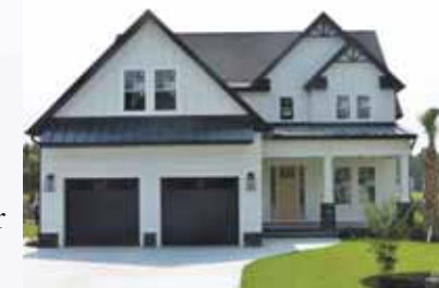
Suncoast Building Products & Services installed the gutters on this home built by MJM Custom Home Building.
