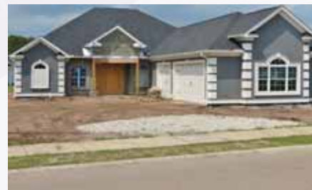
Suncoast Building Products & Services installed the gutters on this home built by Brighton Construction.
