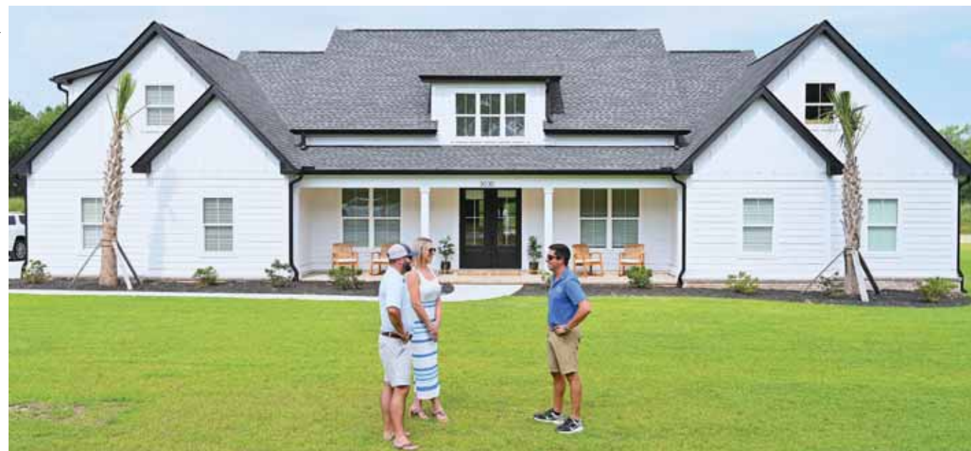
Beach Custom Homes appreciates the project vision and client goals while communicating with them throughout the construction process. Bryan Slattery Jr. (right) talks with homeowners Tyler & Catie Young in front of their home in the Wild Horse community in Conway, SC. “We felt comfortable with Bryan because he’s such a good builder, so we gave him the free reign to make some decisions,” says Tyler.
