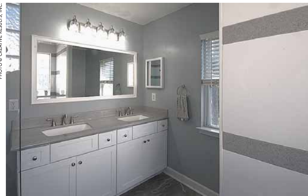
Grey Eastonite vanity top with an integrated white bowl. This is all one piece eliminating any seams.
