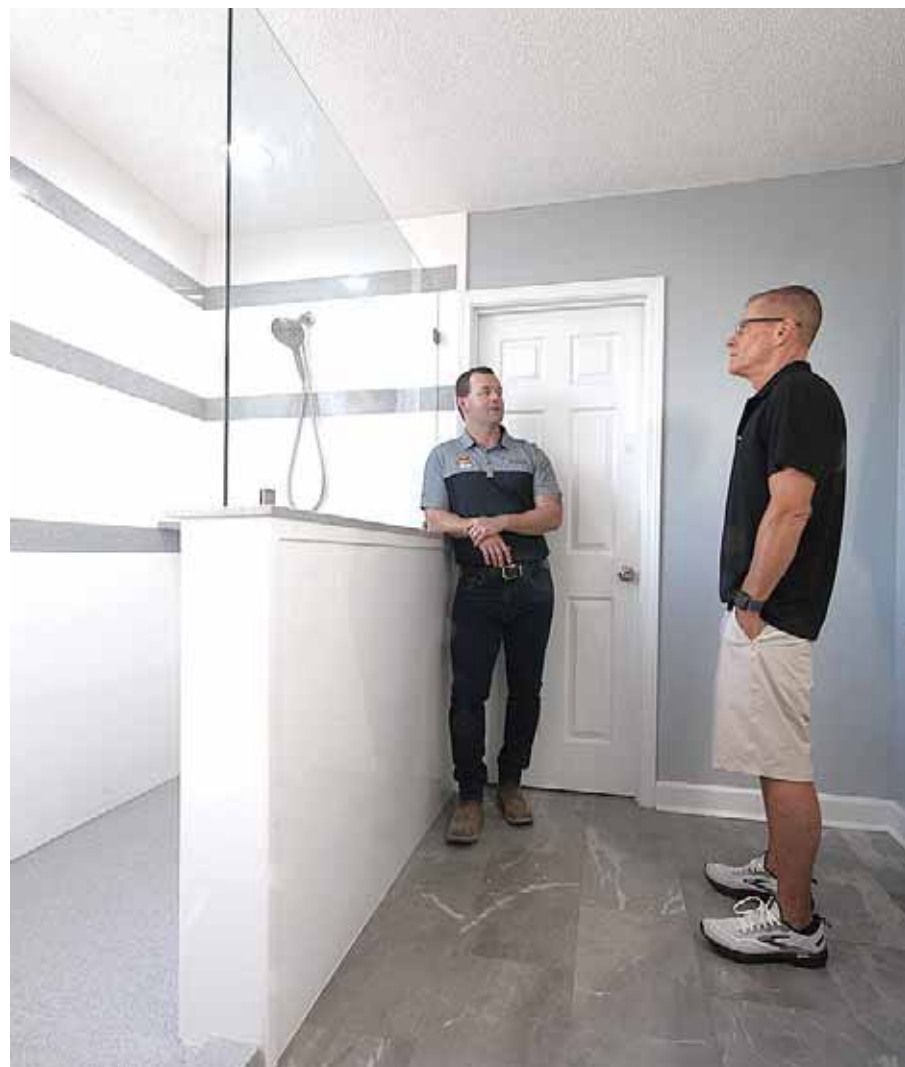
Owner Cullen Marcis ( left ) with the owner of what used to be a tub and shower. That was converted to a massive walk-in shower with white-on-white cultured marble walls and a grey Eastonite inlay and shower pan.
