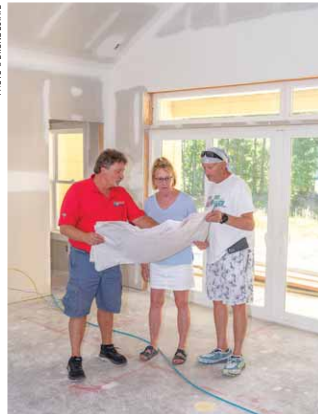
John Lorton (left) with Ronald and Patricia Botti, going over the blueprints of the Botti's new home build to ensure that every aspect of the build is completed to the specifications and satisfaction of the homeowner. The customer's involvement and interaction with the building process ensures their overall satisfaction with the end result.
