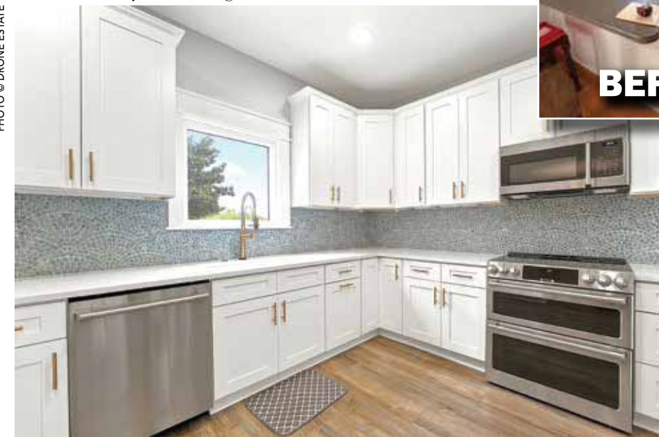
A full kitchen remodel in the Miller residence. The project included new cabinetry, countertops, appliances, custom backsplash, electrical modifications for the undercabinet electrical & recessed lighting, as well as a new window with custom craftsman molding overlooking the pool.
