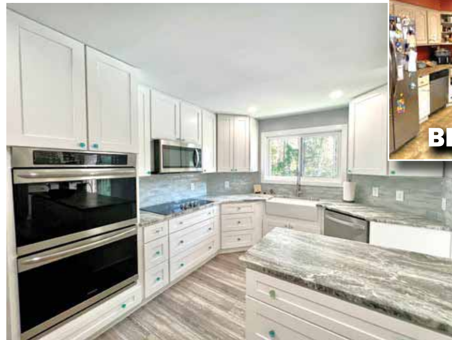
The full kitchen remodel in the residence of Laura Boronski. “They’re awesome! They did three projects for us: gutted our kitchen, remodeled our front and back porches, and they are going to renovate one of our bathrooms, they’re that good. They are 100 percent honest about everything, especially with the budget. They really treat you like family, very prompt, and very polite, which was important to us because we have daughters,” says Boronski.
